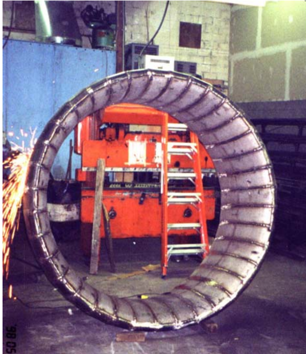
Figure 17. Manufacturing segmented nozzle
