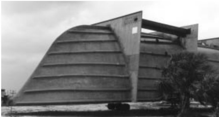
Figure 5-8 Large Female Mold Stored Outdoors at Trident Shipyard [author photo]
