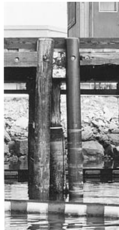
Figure 1-18 Seapile™ Installation as Replacement for Adjacent Timber Pile [Seaward]
