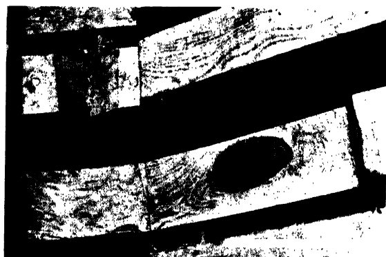
Fig 10. Knot with White Pocket Rot in a floor member
