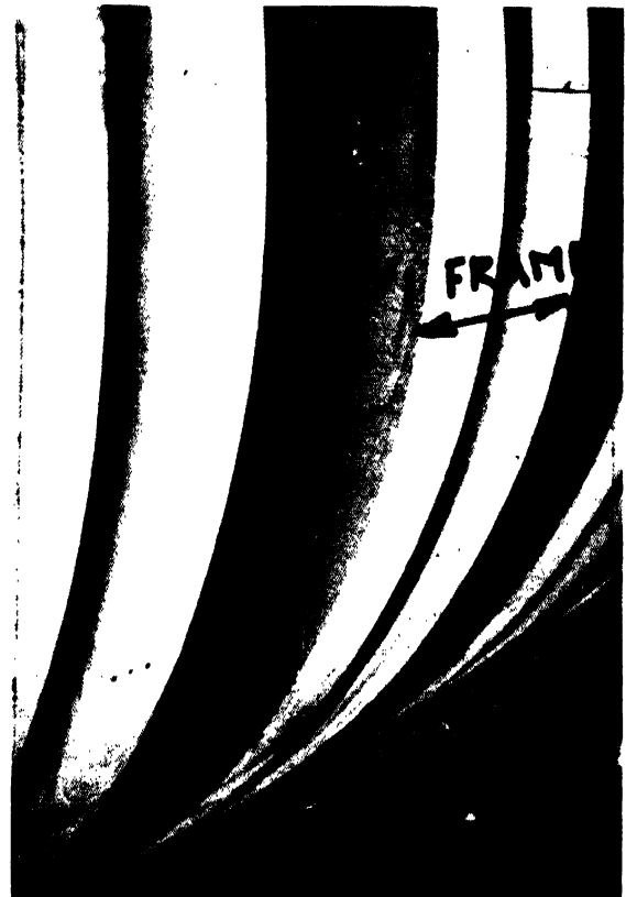
Fig 15. Shake due to cross grain in a frame member
